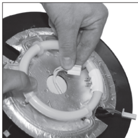
Disconnect the UV-tube.
